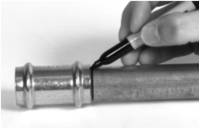
Figure 5 – Marking the Tubing
