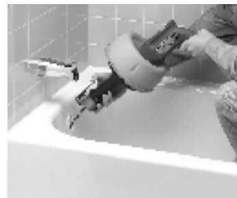
K-39 quickly opens clogged tub lines.
